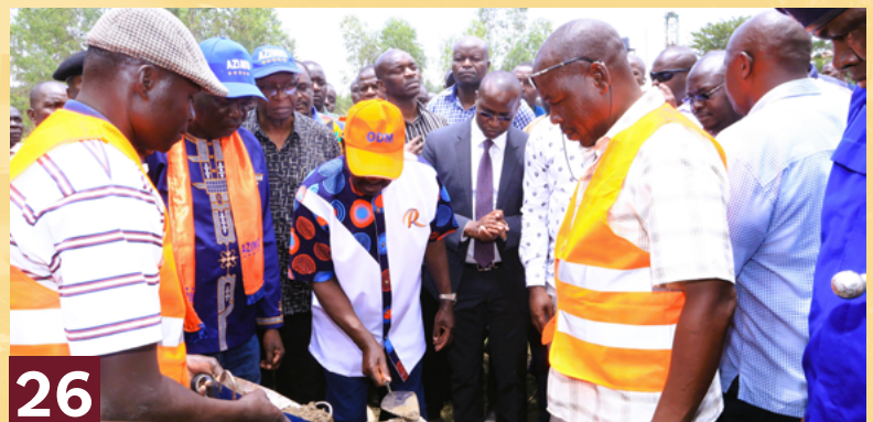
KMTC Students Biggest Winners as College kicks off construction of 300 capacity hostels
