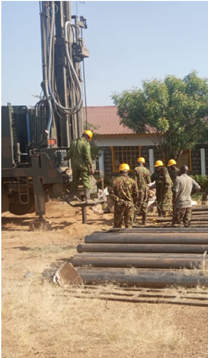
Borehole drilling at Chemolingot Campus.
